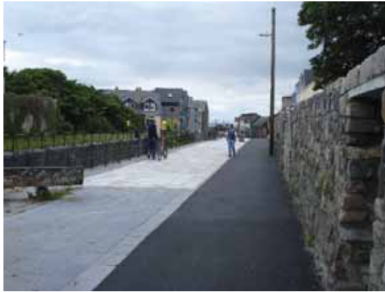
Renovated wall and new footpath along Eglinton Canal
