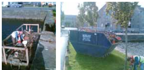
Left: Ongoing maintenance and cleanup of Waterways
