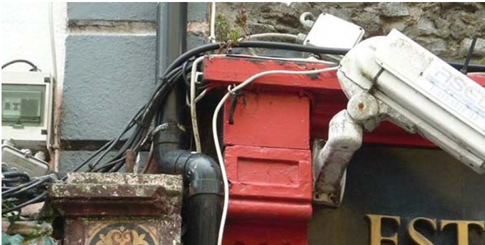
Redundant, excessive, or poor coordinated cabling and services greatly degrades the character of Galway City.
