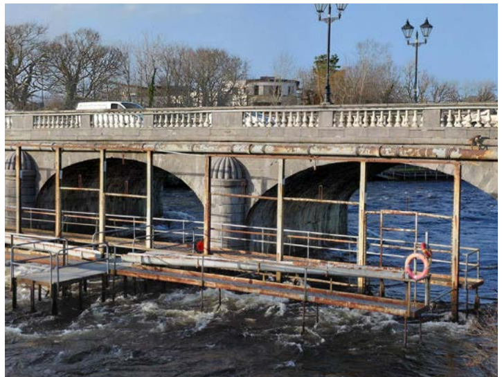
Salmon Weir Bridge showing completed de-vegetation works
