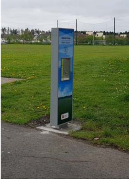
Water station installed at Doughiska.
