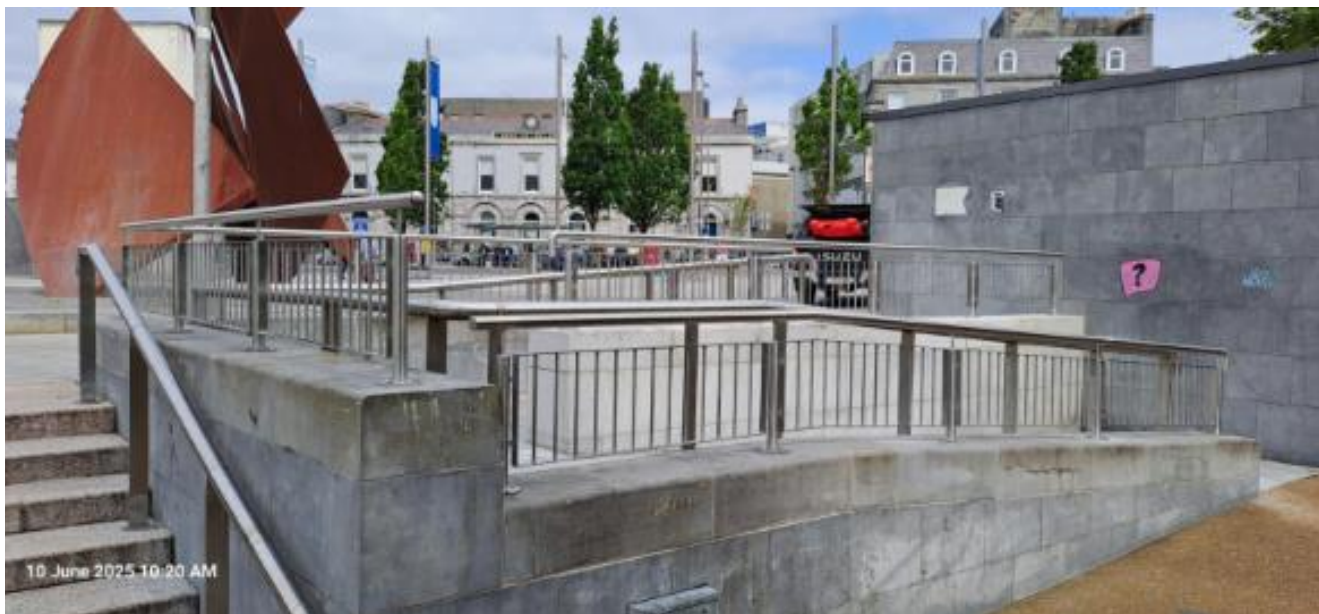
Completed refurbishment works to Eyre Square Pedestrian ramp.
