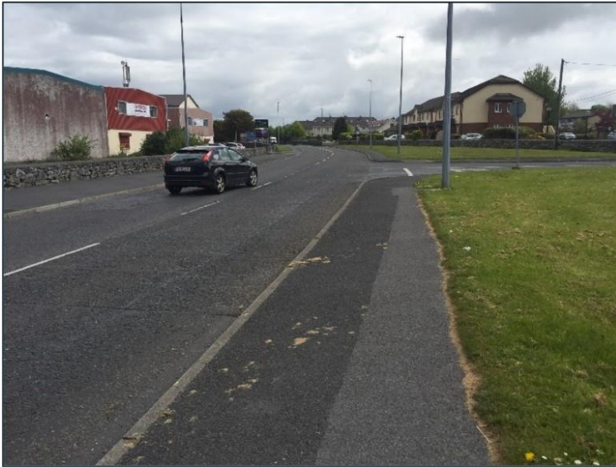
Figure 4-2 - Monivea Road East.
